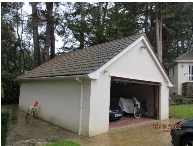
Photo 4: Detached garage in the east.
