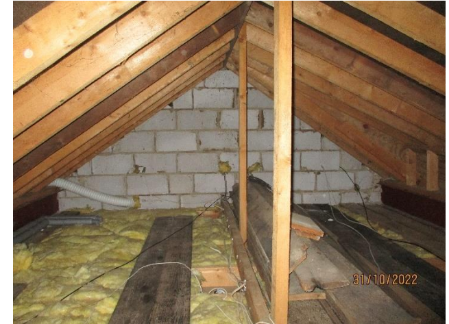
Photo 3: Internal of house loft void.
